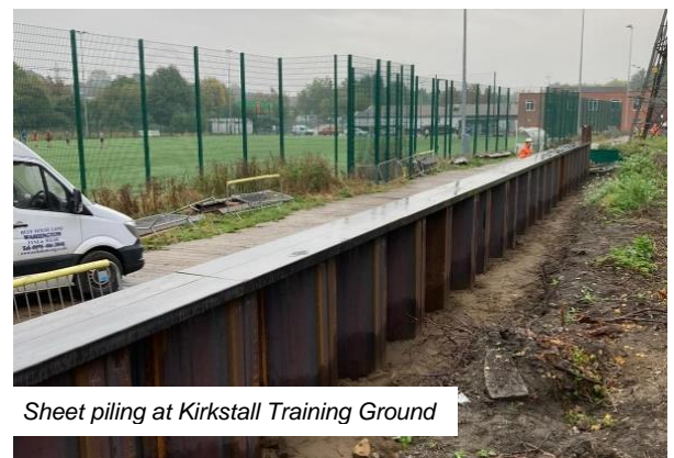
Stone causeway and sheet piling in Zone 12c on Kirkstall Rd
