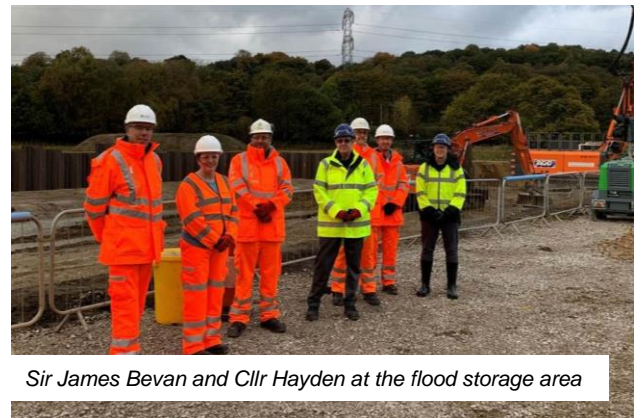
Sheet piling around the cofferdam
